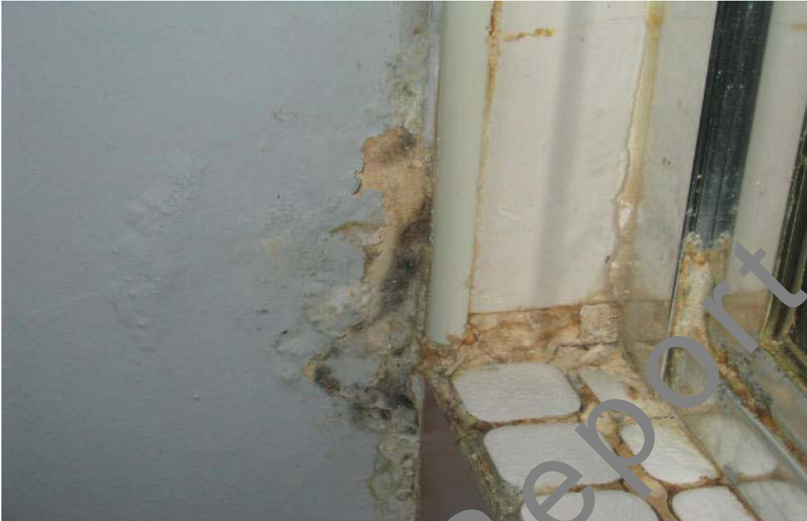
Some prior water damage on the side of the shower wall. Cracks in the shower floor.
