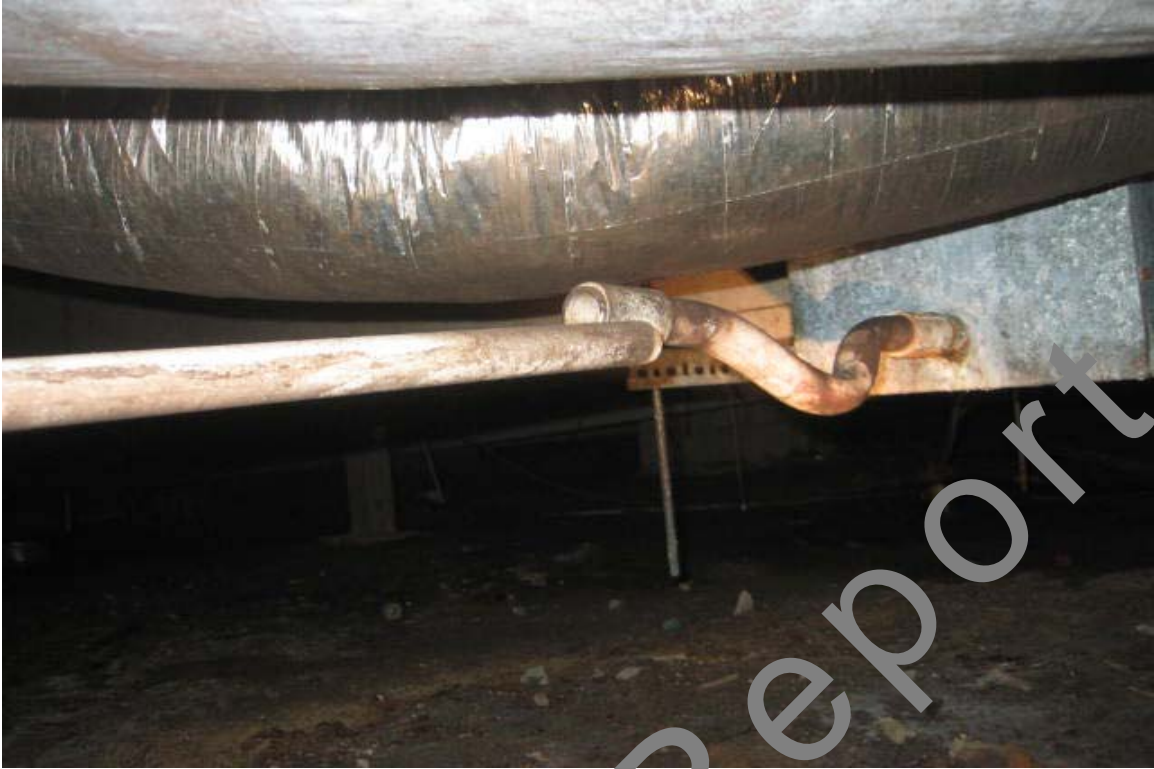
Condensation line has broken. The pipe sticking up on the right side appears to be the way the Jacuzzi is drained.
