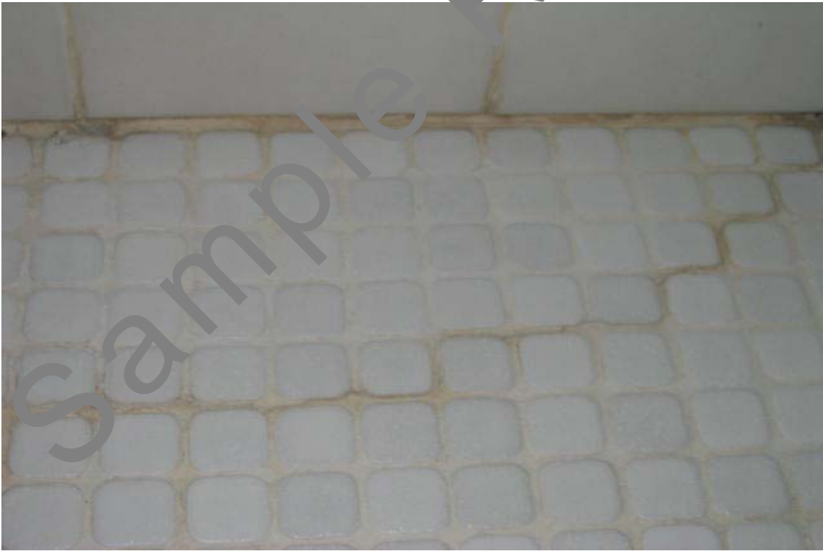
Some prior water damage on the side of the shower wall. Cracks in the shower floor.
