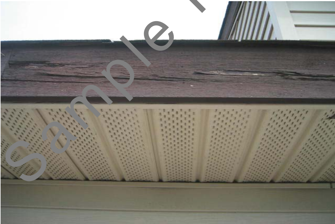
Siding has some exposed nails on the left gable end of main house. Some rot on the rear fascia.
