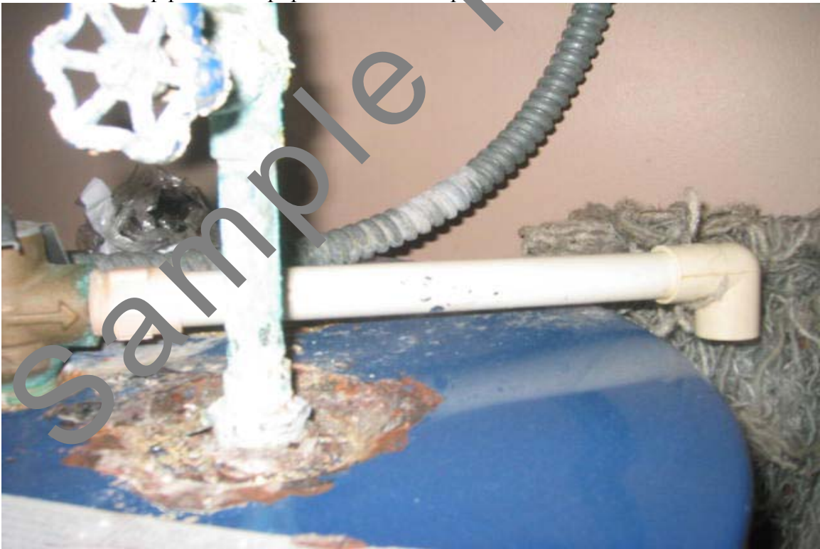
Fixed patio door in the living room is damaged. Rust around the pipe and the pop off valve is not plumbed down.
