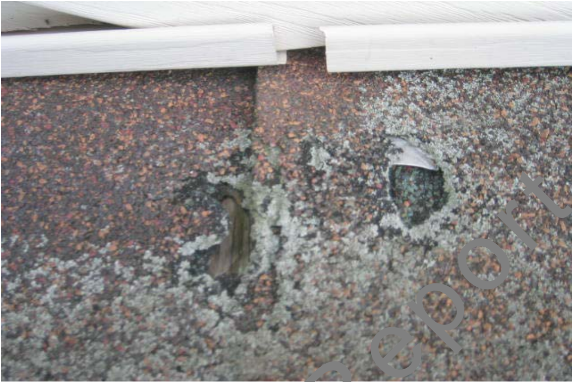
Hole in the roofing shingles on the right side of the house, next to the gable end. Shingles missing on the garage.
