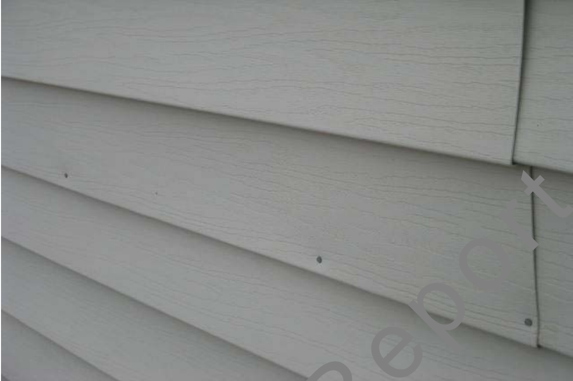
Siding has some exposed nails on the left gable end of main house. Some rot on the rear fascia.
