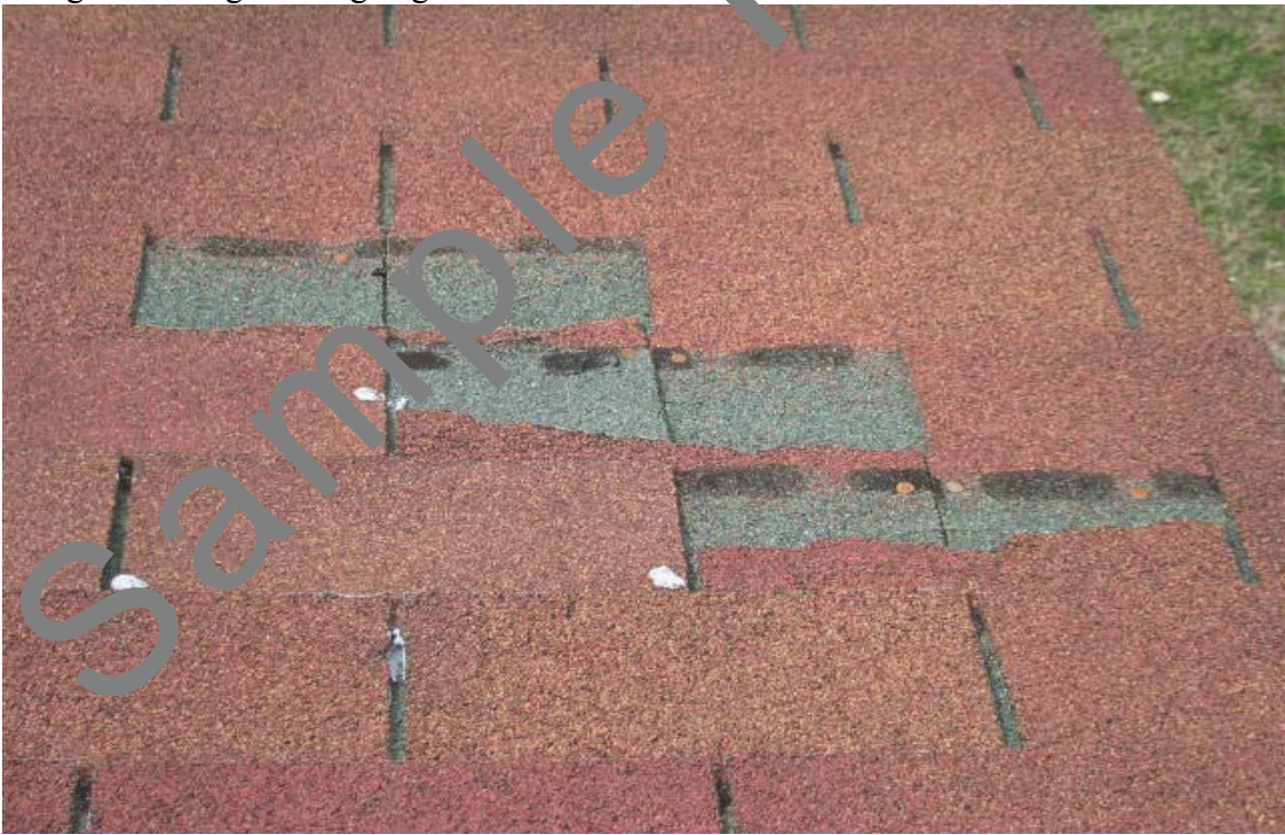
Hole in the roofing shingles on the right side of the house, next to the gable end. Shingles missing on the garage.
