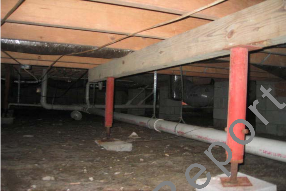
Several temporary jacks under the house to support the span. Furnace under the house.
