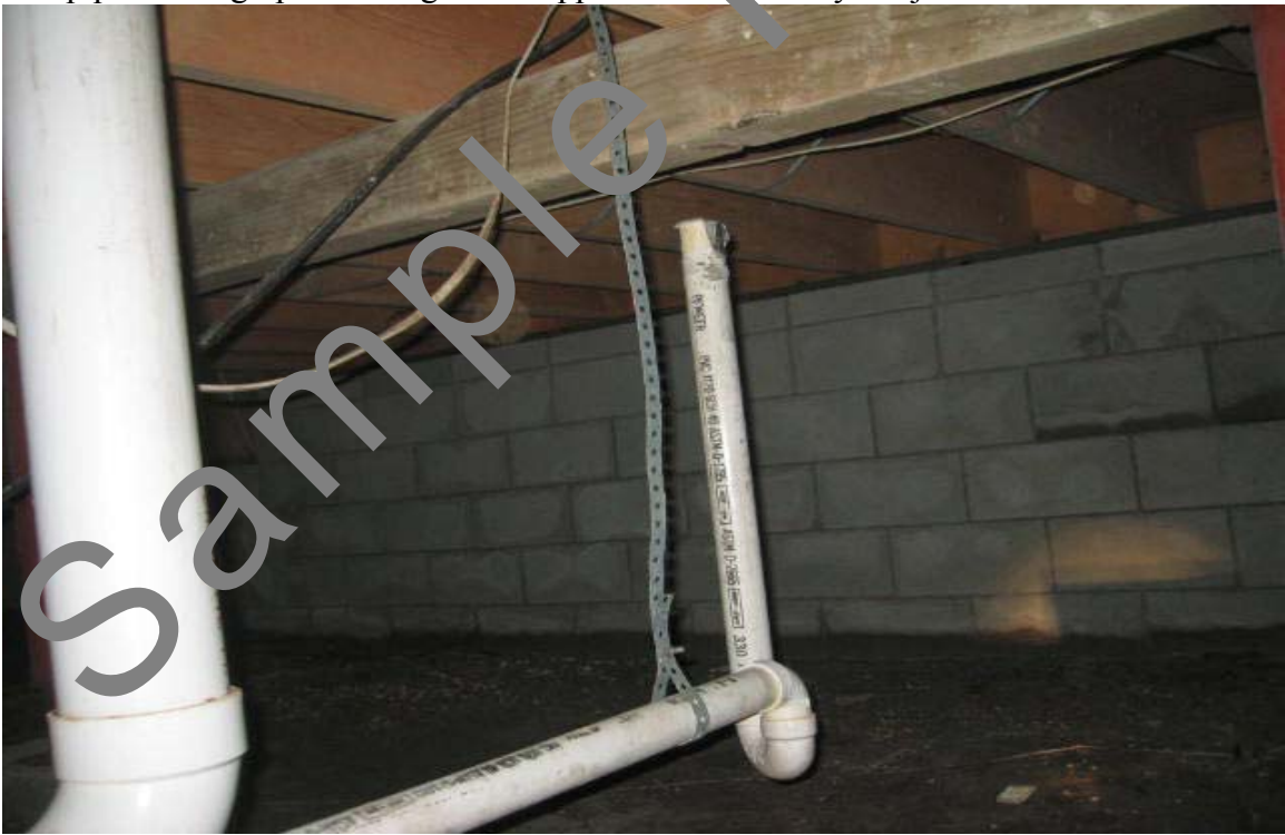
Condensation line has broken. The pipe sticking up on the right side appears to be the way the Jacuzzi is drained.
