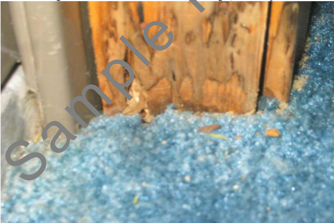
Rust around the bottom of the hot water heater. Some rot damage on the left side of the first room on the right, floor and jamb.
