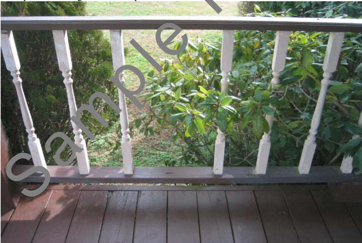
Light fixture cover missing on the front. Rail spindle missing on the front porch.
