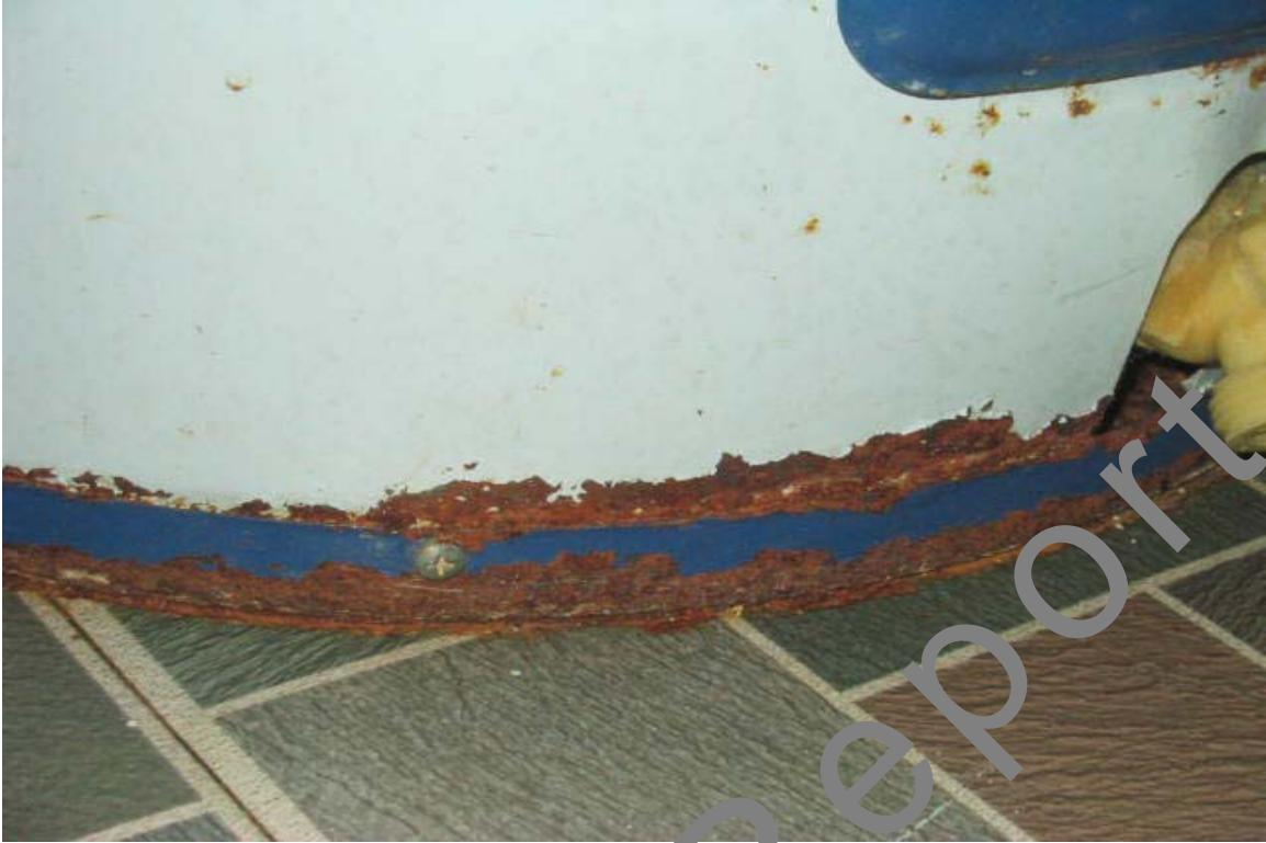
Rust around the bottom of the hot water heater. Some rot damage on the left side of the first room on the right, floor and jamb.
