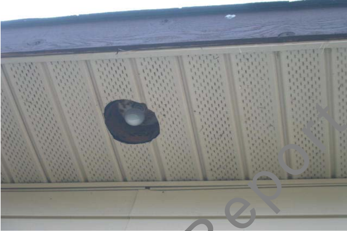
Light fixture cover missing on the front. Rail spindle missing on the front porch.
